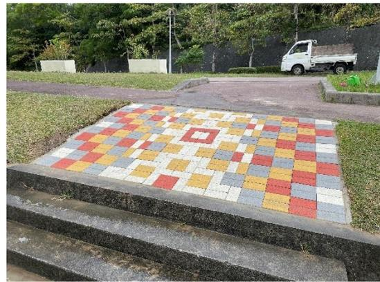
**Figure 3. Construction site after laying interlocking concrete blocks**
