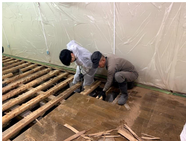
Fig 2. A work in a day as disaster volunteer (Tearing up the floor with a crowbar)
